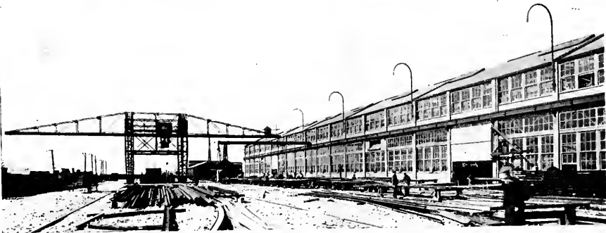
Exterior of the plate shop, showing large traveling gantry for handling material in the plate storage space.
